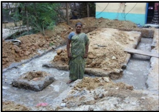
Commencement of Construction
